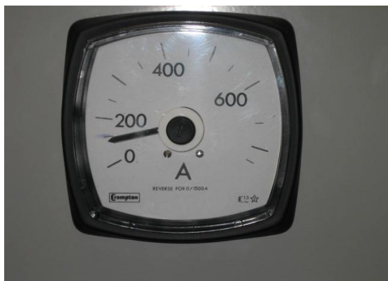
Figure 5 A switchgear ammeter
